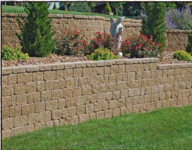
ALIGNMENT WITHOUT PINS FOR LANDSCAPE WALLS
